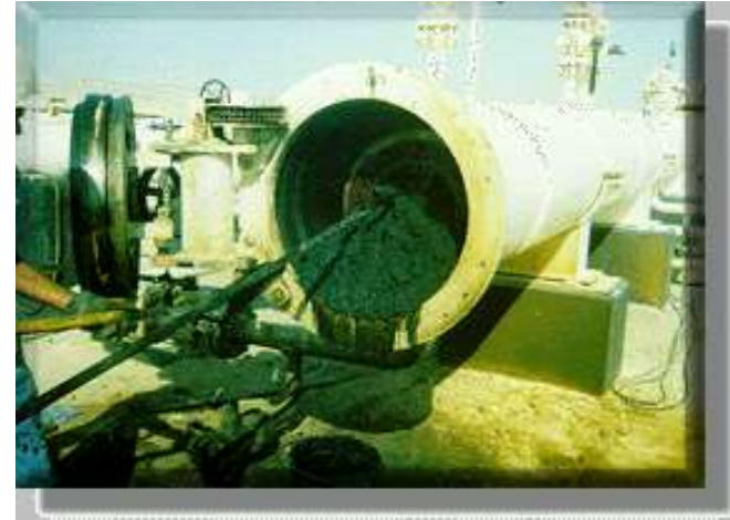
Sand deposition at the flowlines
